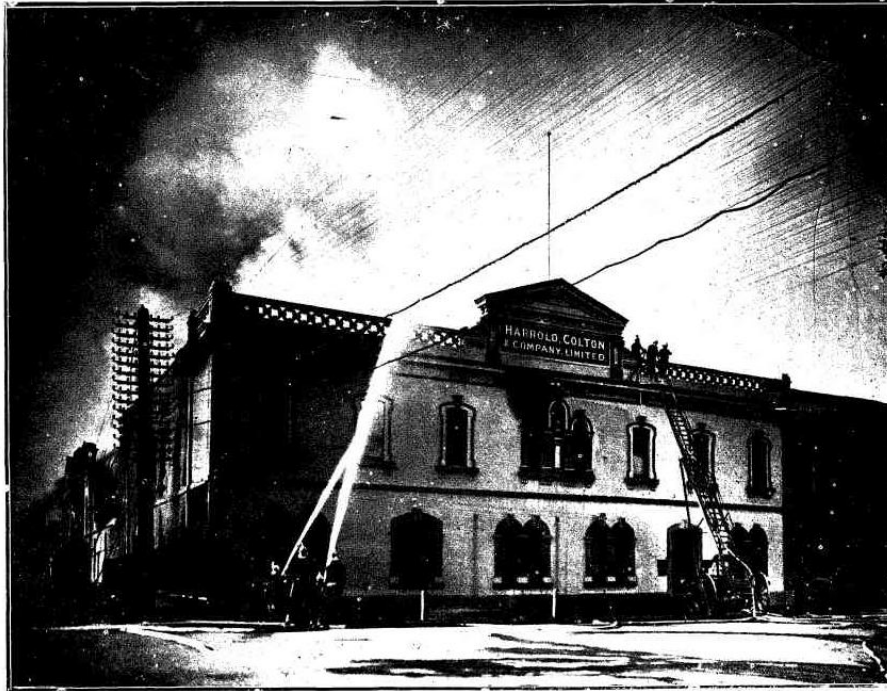
Two Views of the Fire at Harrold, Colton, & Co.'s Premises.
