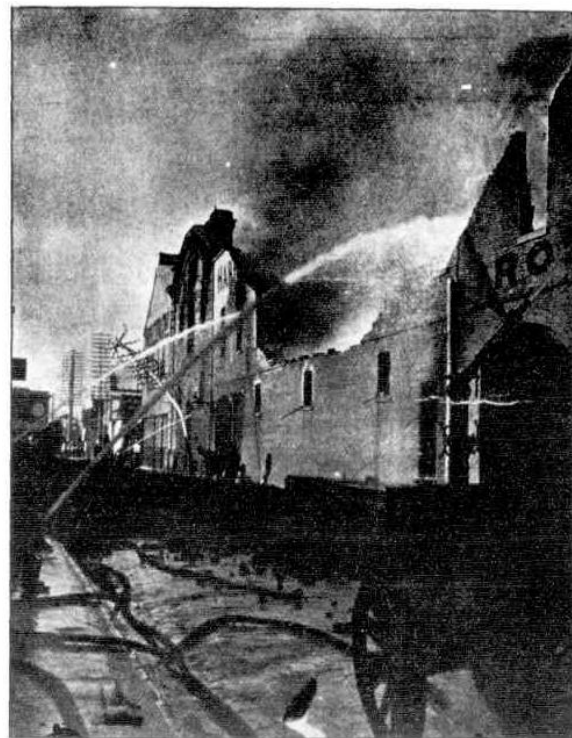
A SUBSEQUENT PICTURE SHOWING THE EASTERN WALL FALLEN AWAY.
